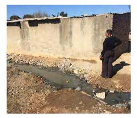
**Figure 4.2:** Erosion causing the undermining and collapse of part of a dwelling
